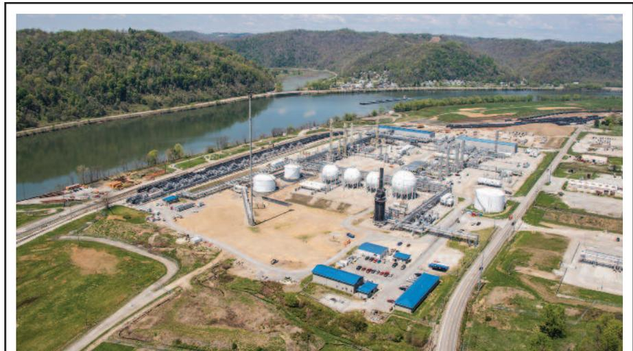
Blue Racer Midstream's Natrium natural gas processing and fractionation facility, which is located on the Ohio River in Marshall County, W.V., has a processing capacity of 400 million cubic feet of natural gas a day. The facility's 123,000 bbl/d fractionator strips the ethane, propane, butane, and natural gasoline from the Y-grade natural gas stream fed into the plant.
